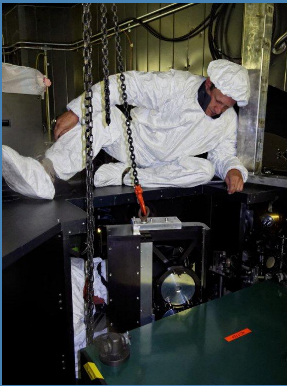
Figure 2. Installing the stage for the dichroic beamsplitters on the AO bench just in front of OSIRIS. ★
