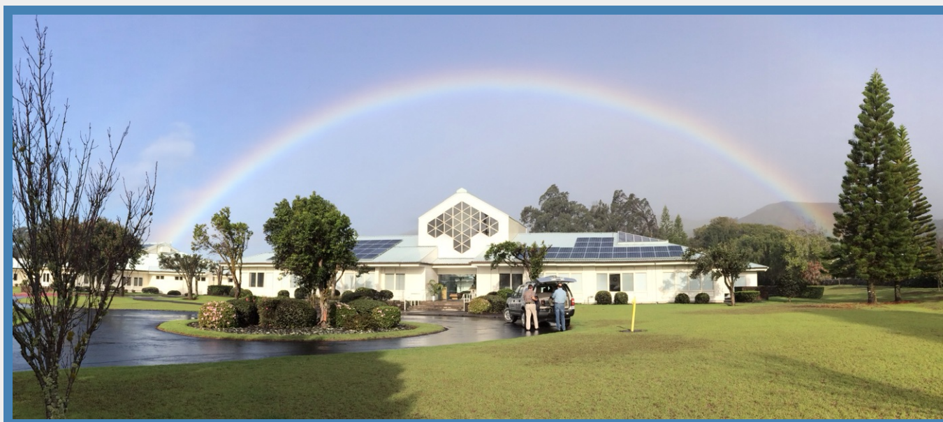
Figure 6. Installation of solar panels on the roof of the Keck Observatory headquarters in Waimea. (Photo: Bob Goodrich)
