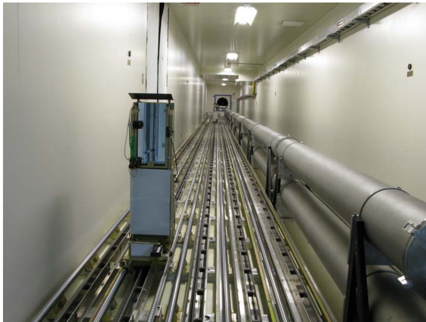
Fig. 3. The quasi-static long delay lines of the Keck Interferometer can correct for \pm 70 m of geometric delay.
